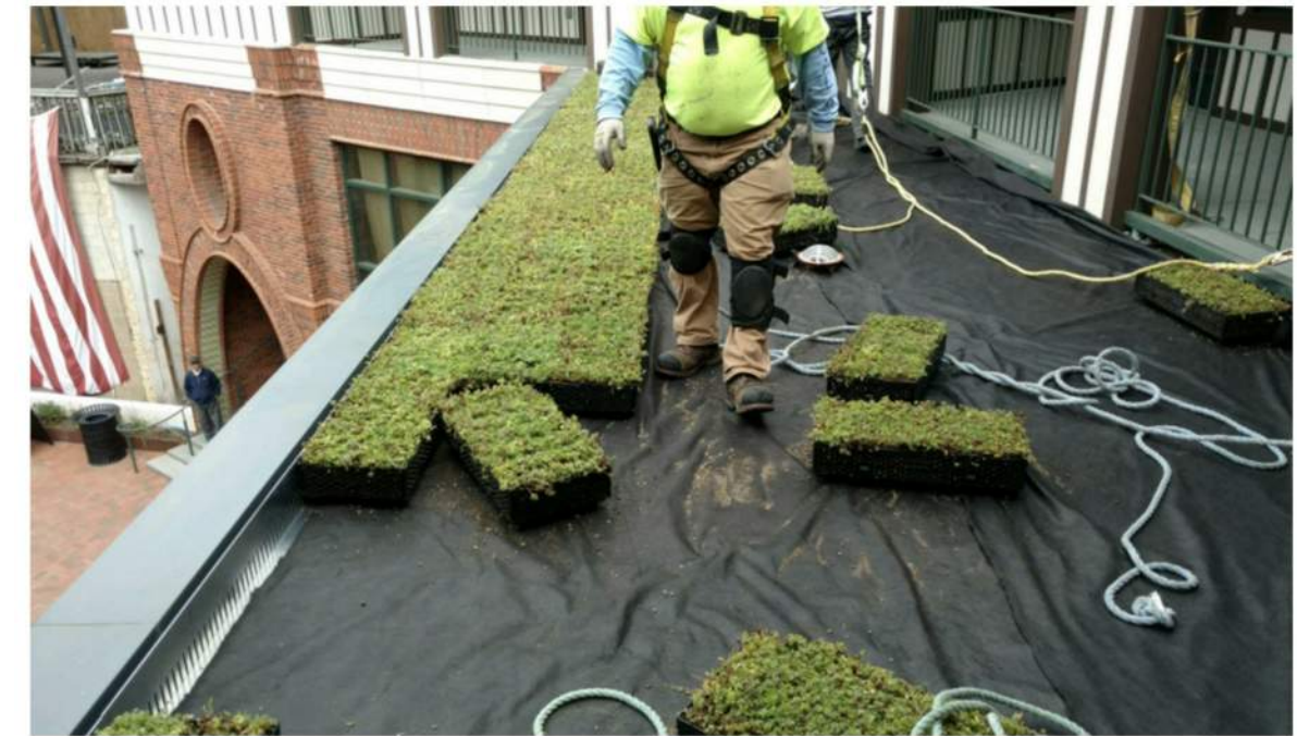
MODULAR PLANT TRAYS GREEN ROOF REFERENCE
